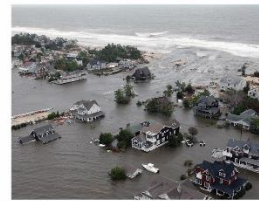
High-tide flooding and increased storm surge
